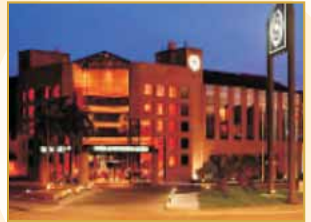
Sheraton Pilar Hotel & Convention Center
